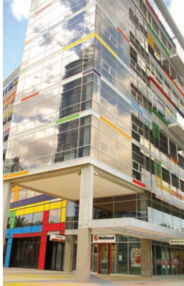
NATIONAL AUSTRALIA BANK AT DOCKLAND - VIC
