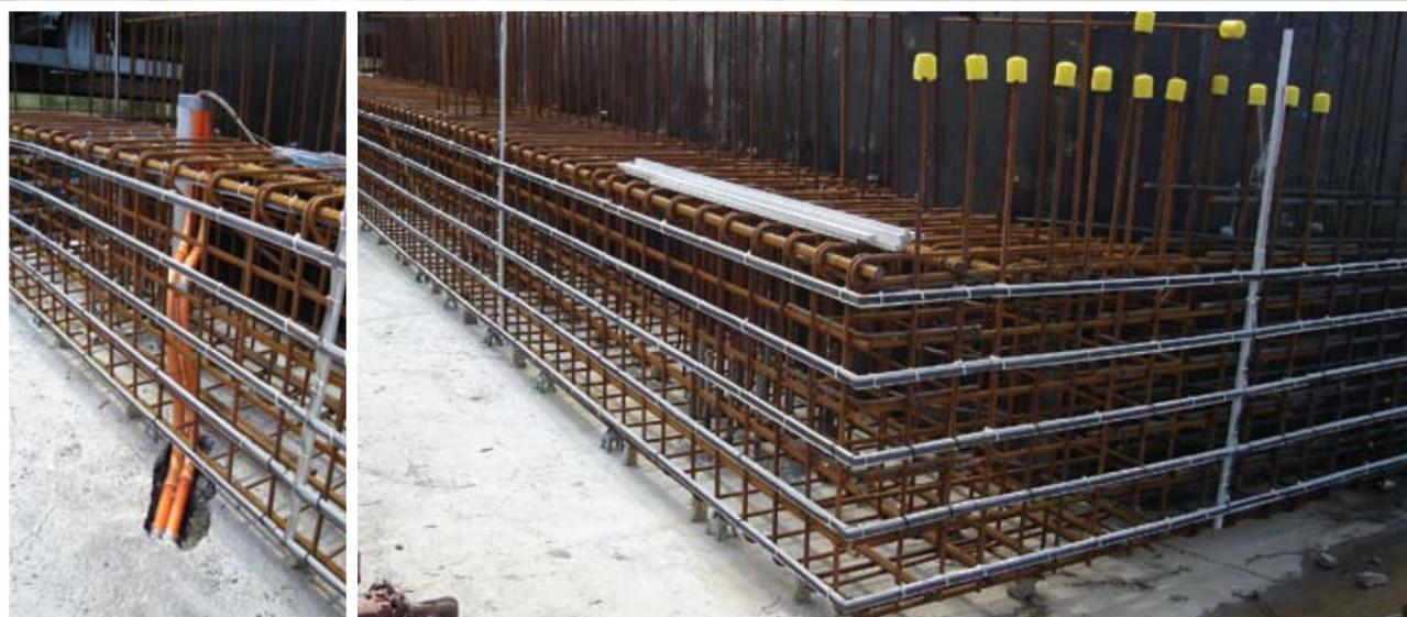
Corrosion Control Engineering (NSW) Pty Ltd were engaged by Daracon Contractors in December 2008 to re-design, supply, install and commission an Impressed Current Cathodic Protection (ICCP) System to the new Tourle St Bridge, which runs over the Hunter River in Mayfield, Newcastle.
