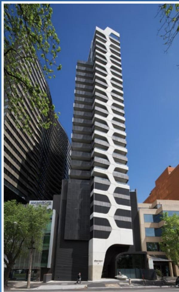
The spectacular curved precast lattice on the facade of Albert Tower makes it obvious that this was a challenging project, requiring a high level of creative thinking to deliver the design by Architect Rothe Lowman. For Icon Construction Australia (Icon Co), resolving the implicit constructability puzzles of this remarkable 30-level tower resulted in a tremendous demonstration of innovation in action.
