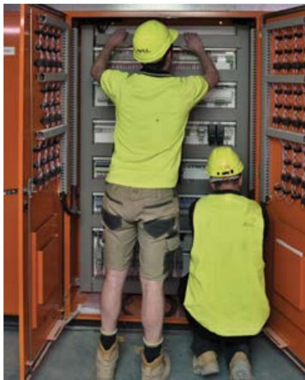
Pope manufactured a pressurisation control system with four pressurisation fans which controlled the central pressure of the stairwell, as well as regulating two smoke spill exhaust fans. "The system used ABB variable speed drives, the Eliwell system and four Dwyer static pressure transducers," Bradley said.
