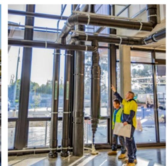
**Below** Geothermal Industries Australia (GIA) drilled 28 vertical bores and installed 2,500m of energy pile piping.
