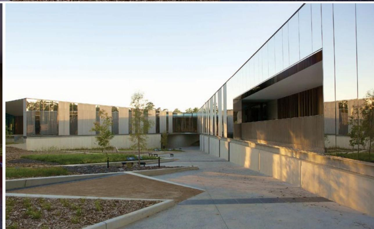
The building finishes are feature elements, some of which have been constructed for the first time in Australia including the stainless steel mirror panel façade and 4.5 metre toughened curved glass panels. Colour controlled concrete walls with blow holes and landscape walls that splay and change direction in a series of triangulations add to the three dimensional illusions in the building.
