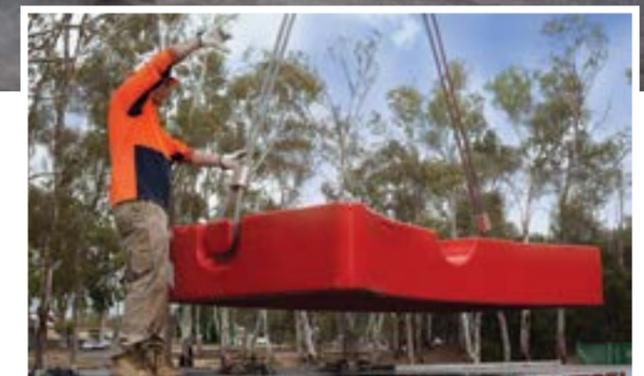
an active construction site, with multiple obstacles, such as high voltage power-lines, other trades, plant and machinery are challenges we frequently encounter. Our pre-site analysis, development of a SWMS and Lift Studies guided us in selecting the relevant equipment, personnel and work methods suitable for this high-risk work. A specialised lifting method using a 46m spreader bar was used to securely support, lift and place the load.”
