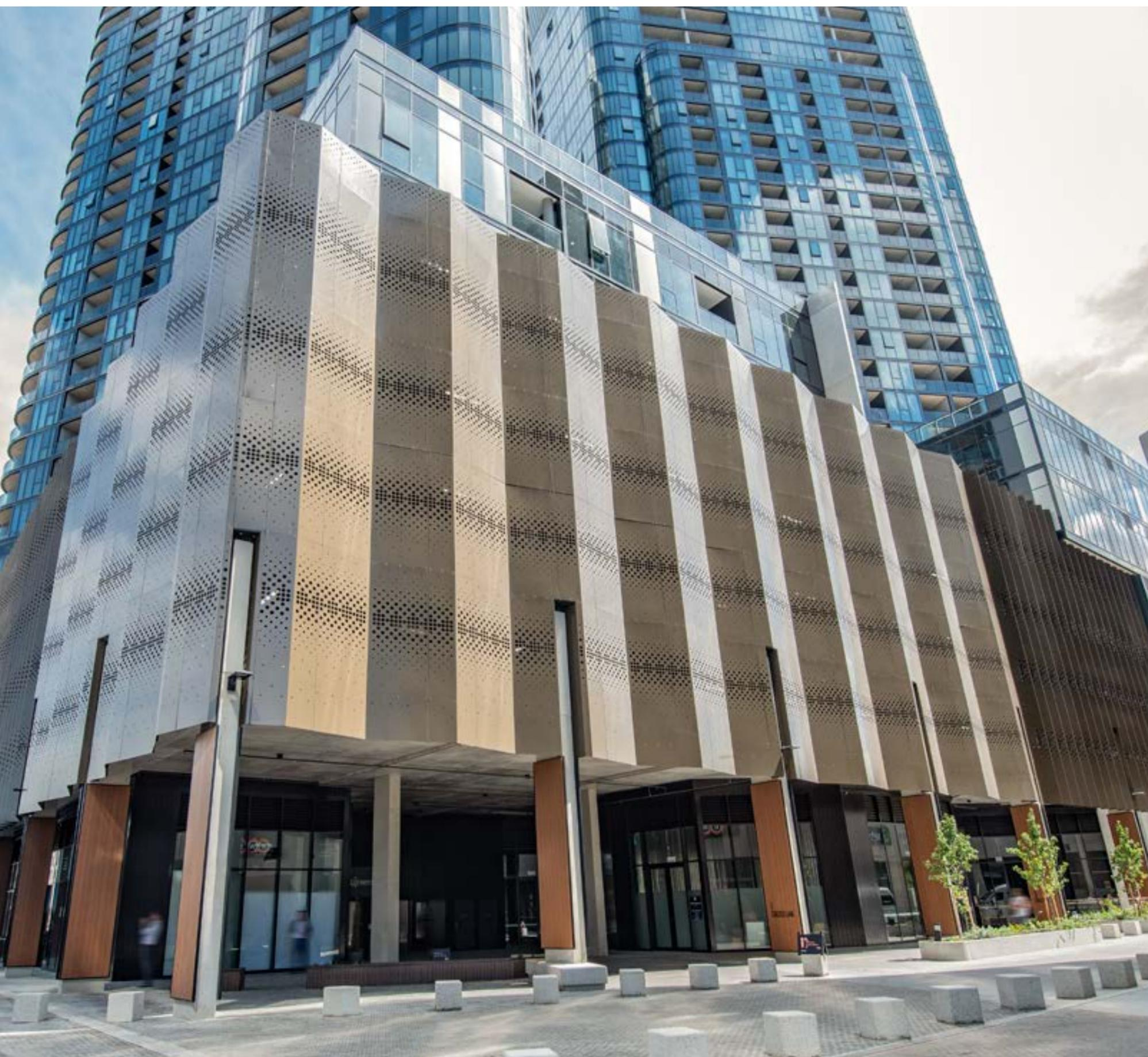
**Renrow Steel design, fabricate and install steel and aluminium elements including structural steel members, stylish façade screens and stunning architectural feature pieces.** In late 2019, Renrow Steel procured and completed design works of 2,200m<sup>2</sup> of aluminium screens for the car park façade of High Society as well as the balustrades to Levels 5 and 23.
