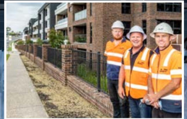
**Three-storey Flemish bond brickwork, nearly 1km of external fencing with brick piers every 2.4m and a common ground package including retaining walls, access ramps and garden beds are just some of the brickwork features at Ryman Healthcare's John Flynn village.**
