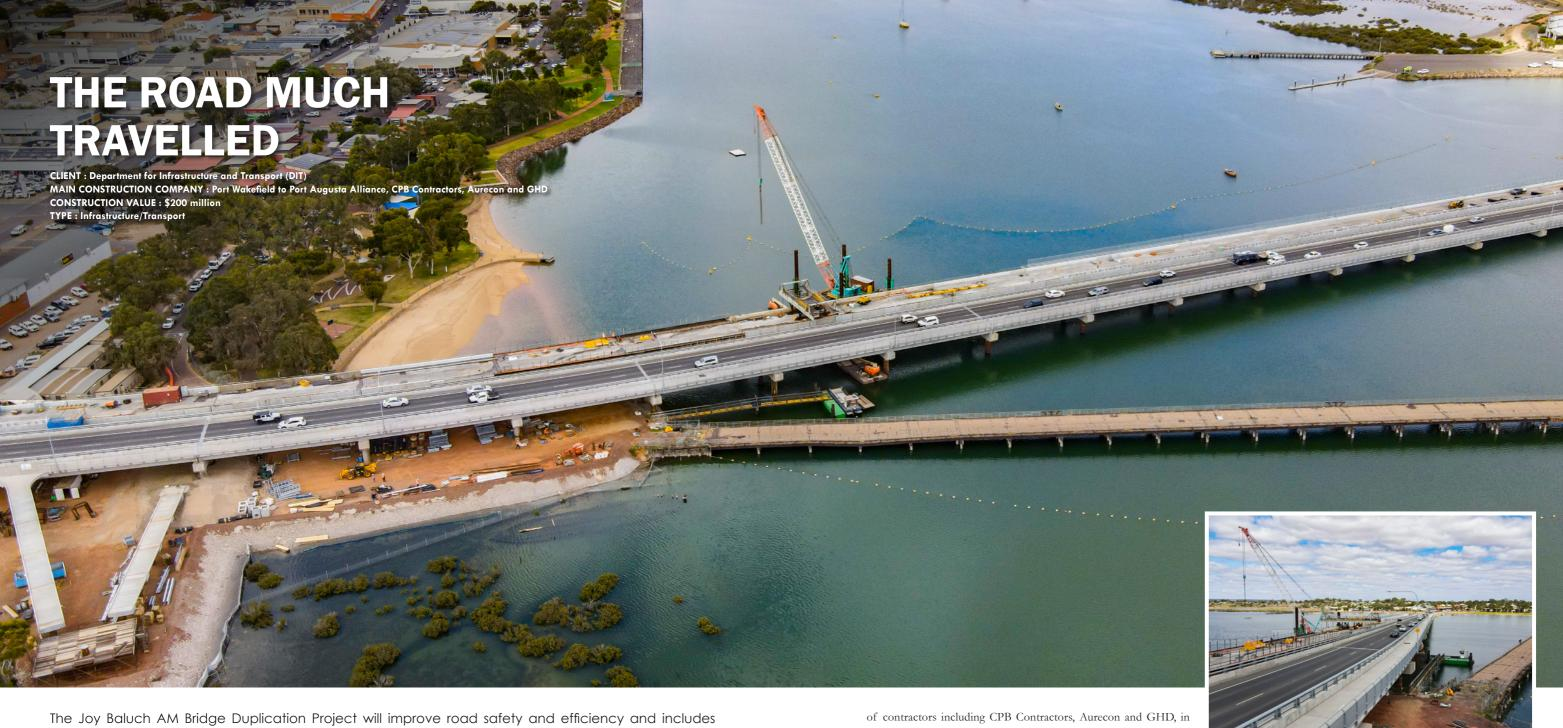
The Joy Baluch AM Bridge Duplication Project will improve road safety and efficiency and includes improved bridge access, new shared use paths, an upgraded intersection at Mackay Street, remediation work and new connections for pedestrians and cyclists.
