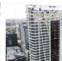
Wrap Apartments Southbank
