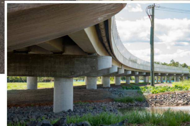
Despite its relatively short distance, more than 170 bridge girders were required for the project, over 10,000m<sup>3</sup> of concrete was poured to build the bridges, and 23,000m<sup>3</sup> of specialised road base was placed.
