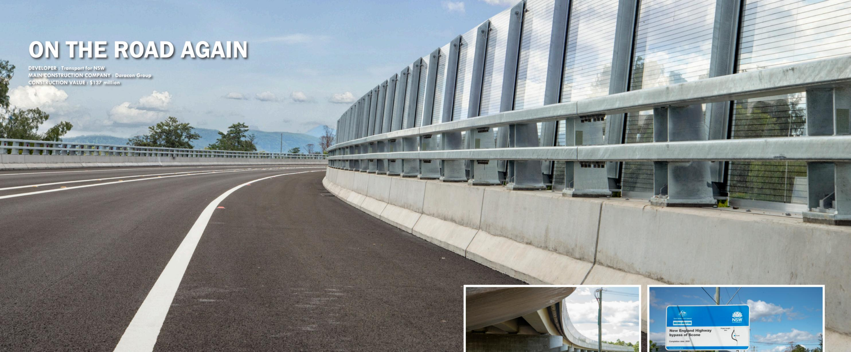
Scone Bypass involved construction of a 5km two-lane bypass which included three new bridges, intersections, associated stormwater drainage, street lights, and road signage. The bypass removes approximately 500 heavy vehicles per day from Kelly Street, and improves road safety and travel times for freight.
