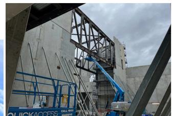
"For this project, we had onsite a 130-tonne, 160-tonne, 220 tonne and 250-tonne mobile crane, a 15-tonne Franna crane, crawler cranes for installing the cladding, various EWPs and a semi with a long trailer to transport the cladding from the factory to site," said Joel.
