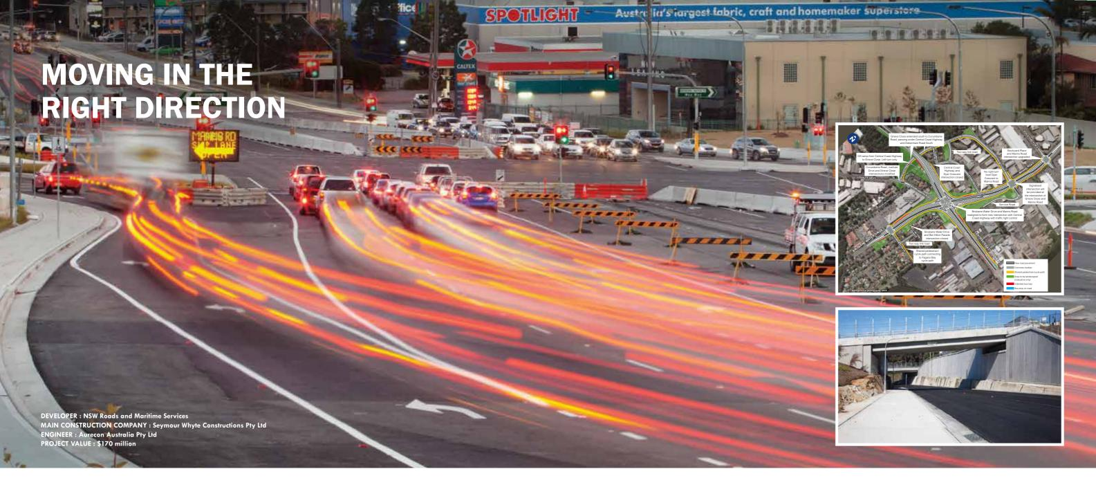
The \$170M Central Coast Highway upgrade has realigned the existing intersection into a single signalised intersection easing congestion. The upgrade included the construction of a new connecting road and a system of shared pedestrian and cycle paths.
