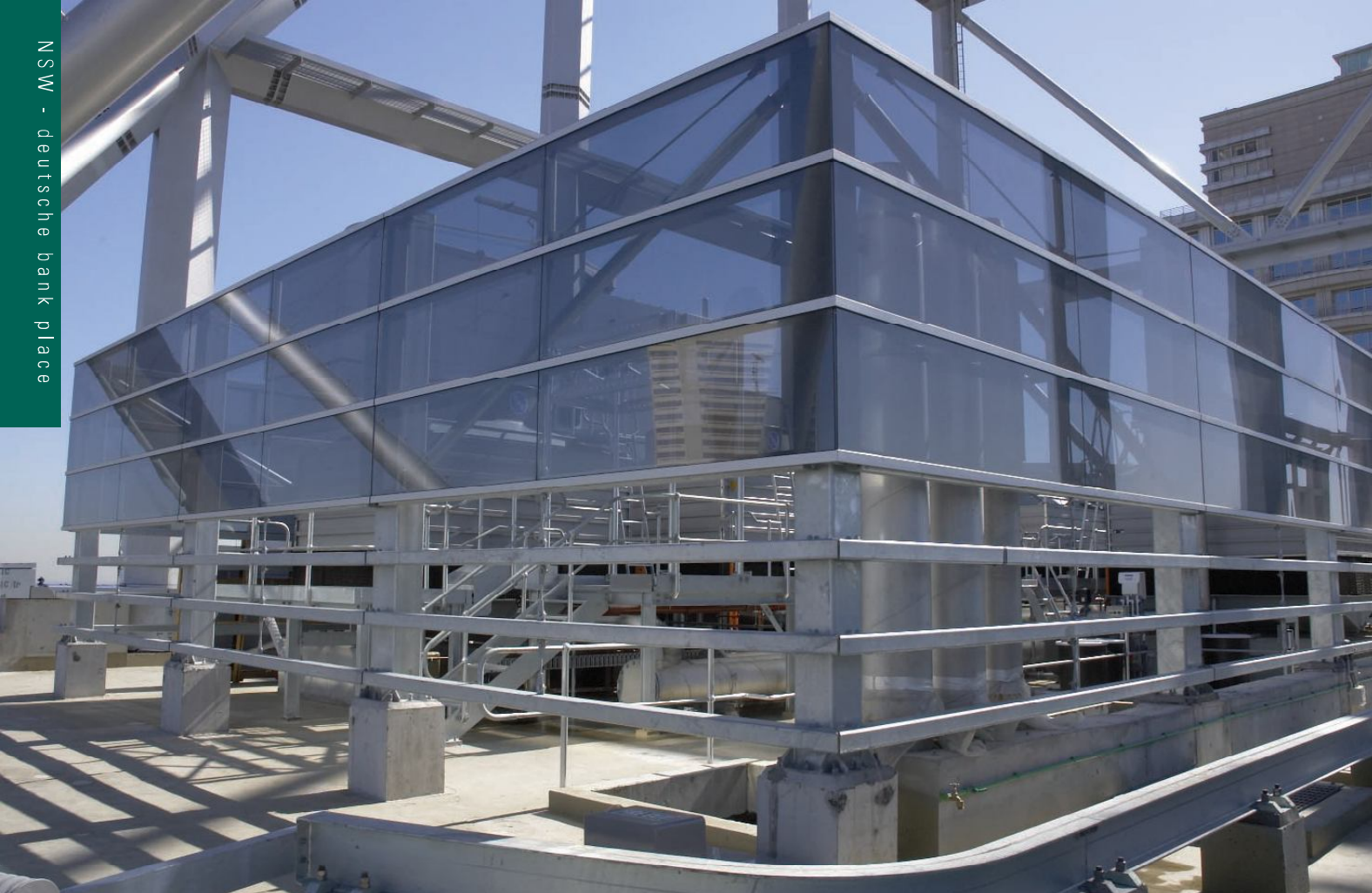
Cooling Tower Enclosure
