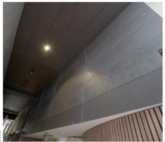
"Diversaclad is a designed system of interlocking panels with mechanical fixings to battens," said Owner, Nick Dong. "The installation required proper planning to build a sub frame and battens onto concrete walls."
