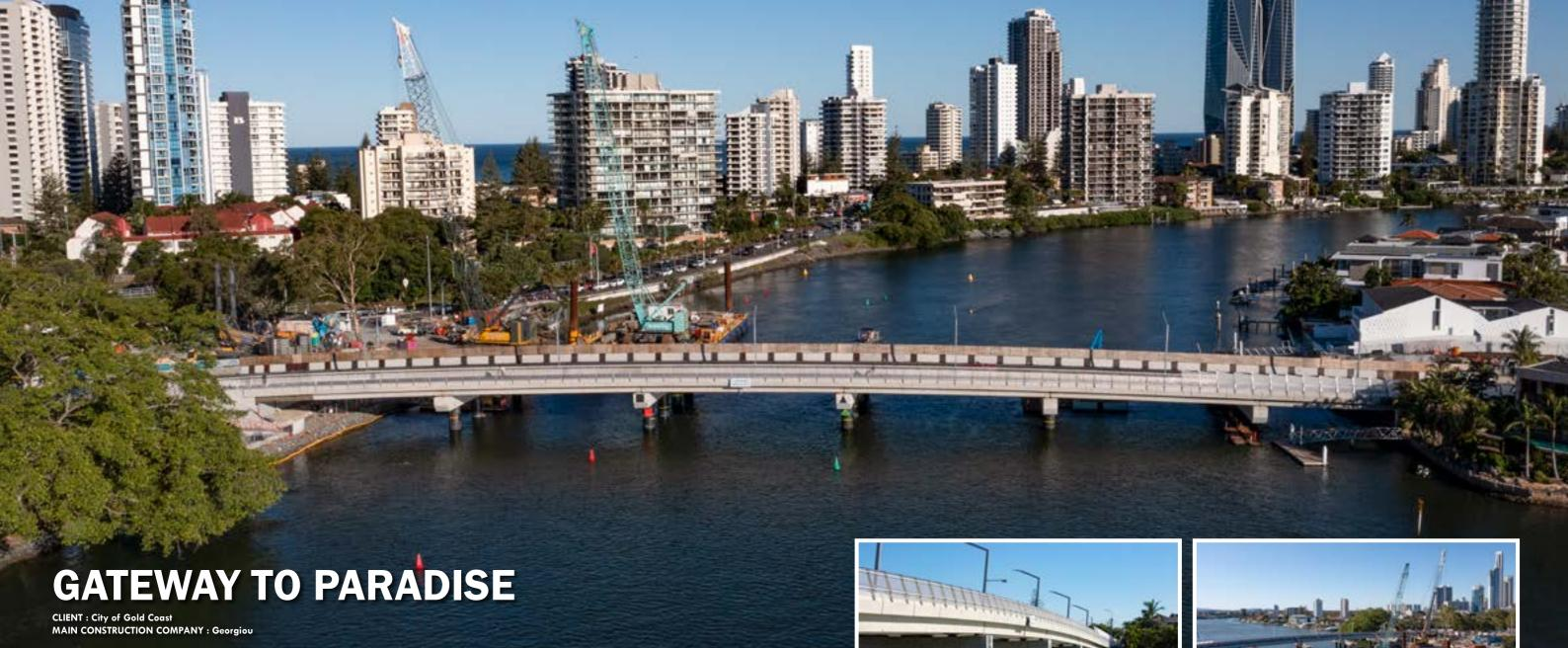
The Isle of Capri Bridge project included the construction of a new 4-lane bridge with an increased clearance height and shared paths on both sides, as well as intersection upgrades on Via Roma and Remembrance Drive, new road connections and improvements to allow for an increased capacity of 25,000 cars per day and reduce congestion.
