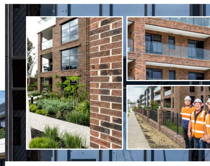
Three-storey Flemish bond brickwork, nearly 1km of external fencing with brick piers every 2.4m and a common ground package including retaining walls, access ramps and garden beds are just some of the brickwork features at Ryman Healthcare's John Flynn village.
