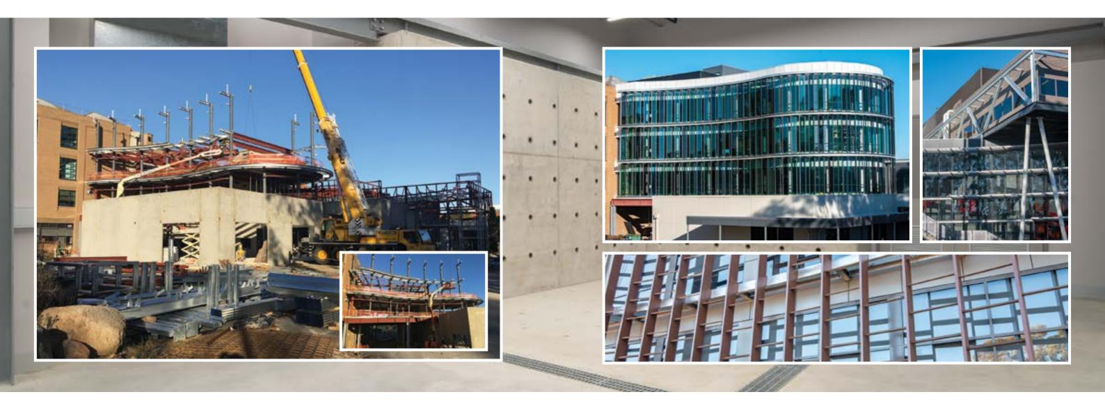
Using the latest technology, to ensure optimum accuracy, SA Structural provided structural steel for the Library at the La Trobe University Bendigo Campus. Having worked with some of the most challenging structures, SA Structural were well equipped to work with the curved façade on this project. The team fabricated and painted the steel at their manufacturing plant before transporting the steel to campus. The highly experienced site crew then carried out the installation.
