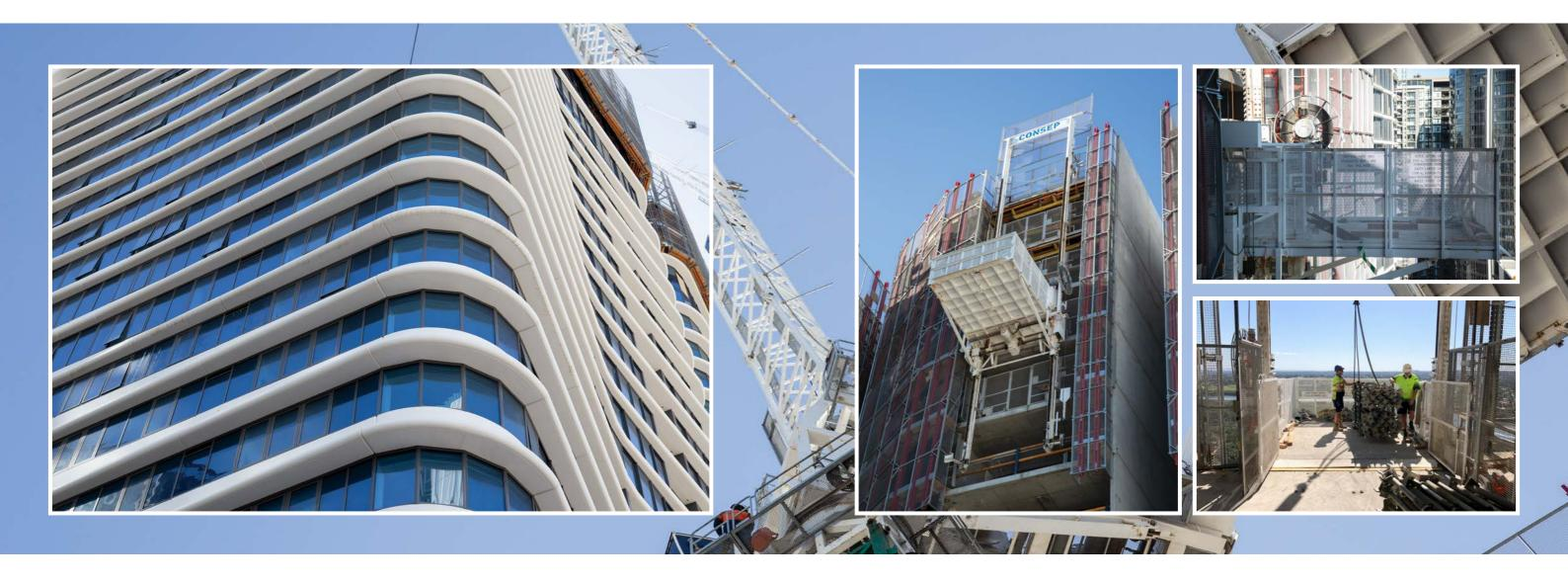
Precast Elements provided the Marina Square Project a total of 4,200 precast panels, balustrades, walls and columns, that were manufactured, installed and finished in all four buildings in varying shapes and sizes, ranging from 200kg to 12 tonne.
