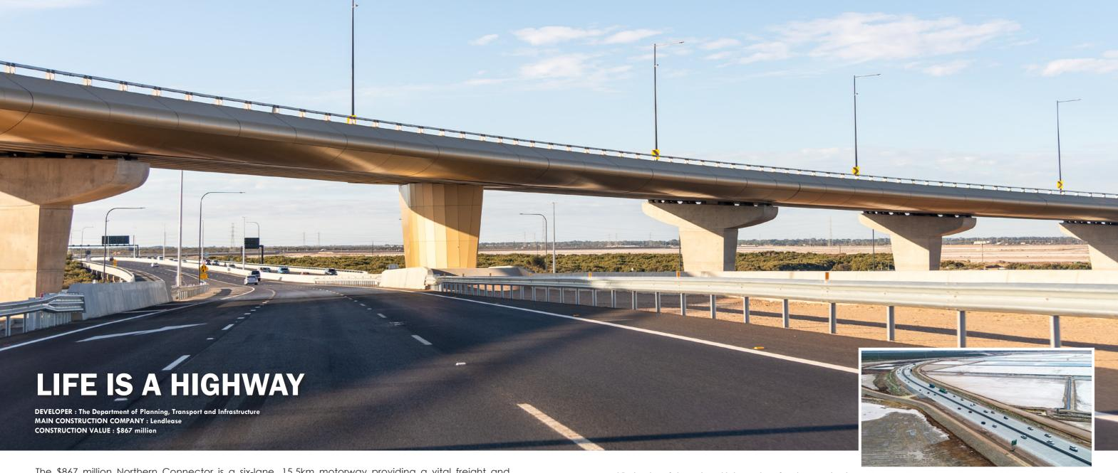
The \$867 million Northern Connector is a six-lane, 15.5km motorway providing a vital freight and commuter link between the Northern Expressway, South Road Superway and Port River Expressway. Predominately constructed from concrete, with a diamond groove finish, the new road took three and half years to complete.
