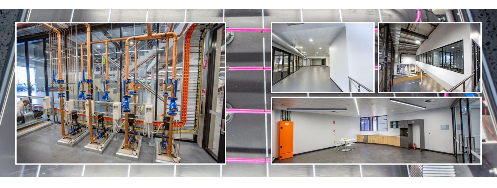
A major contributor to the PICAC Narre Warren project was GeoExchange Australia. They designed, supplied and installed a ground source heat pump (GSHP) system for the heating and cooling requirements of the centre.
