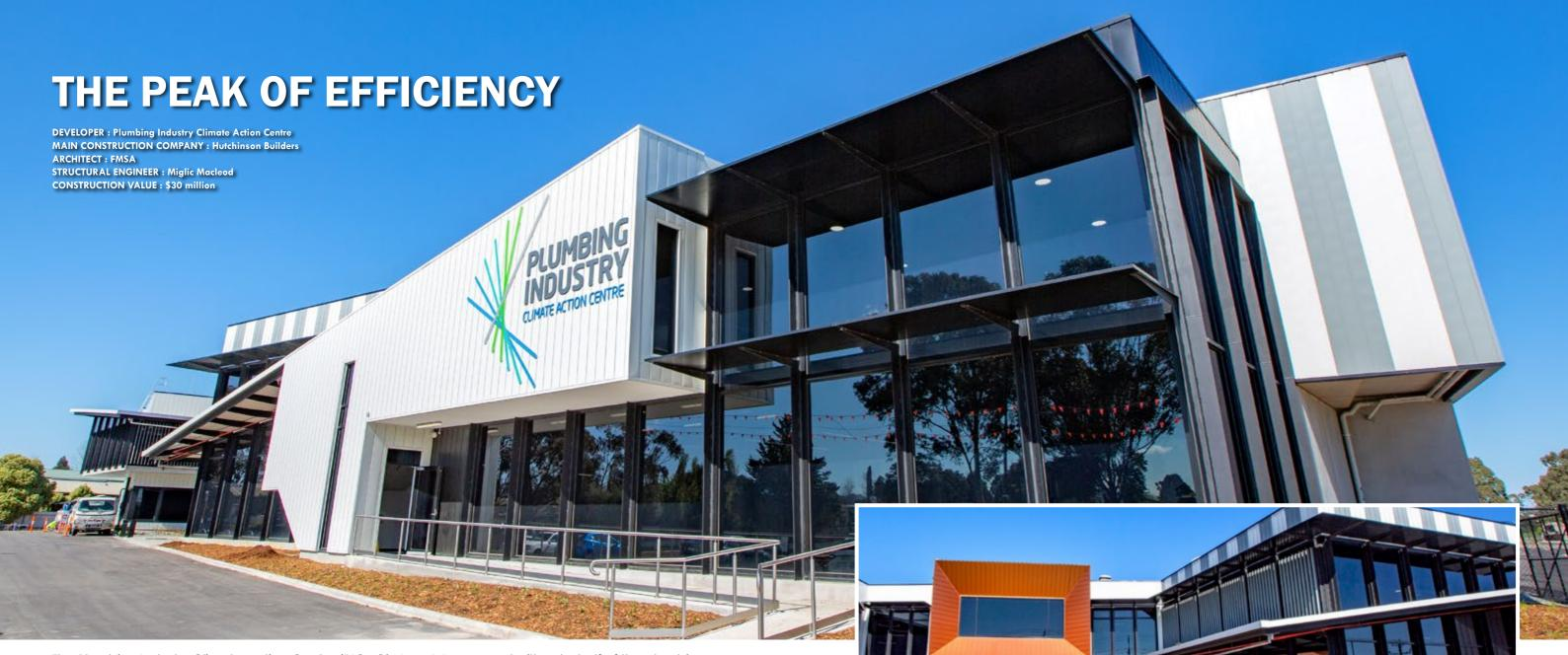
The Plumbing Industry Climate Action Centre (PICAC) Narre Warren was built on behalf of the plumbing, fire protection and HVAC industries, to train plumbing and HVAC apprentices, and pre-apprentices. The building includes a ground source heat pump – closed loop geothermal system with integrated hydronic heating, and thermomass precast panels to ensure a net zero energy rating is achieved.
