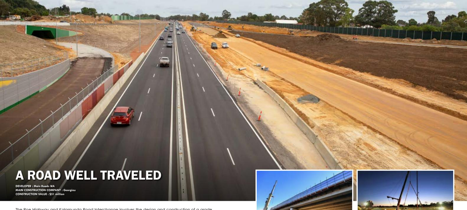
The Roe Highway and Kalamunda Road Interchange involves the design and construction of a grade separated intersection which includes a new bridge, roundabouts, on and off ramps, a shared path for pedestrians and cyclists, along with other supplementary works, and provisions for future extensions.
