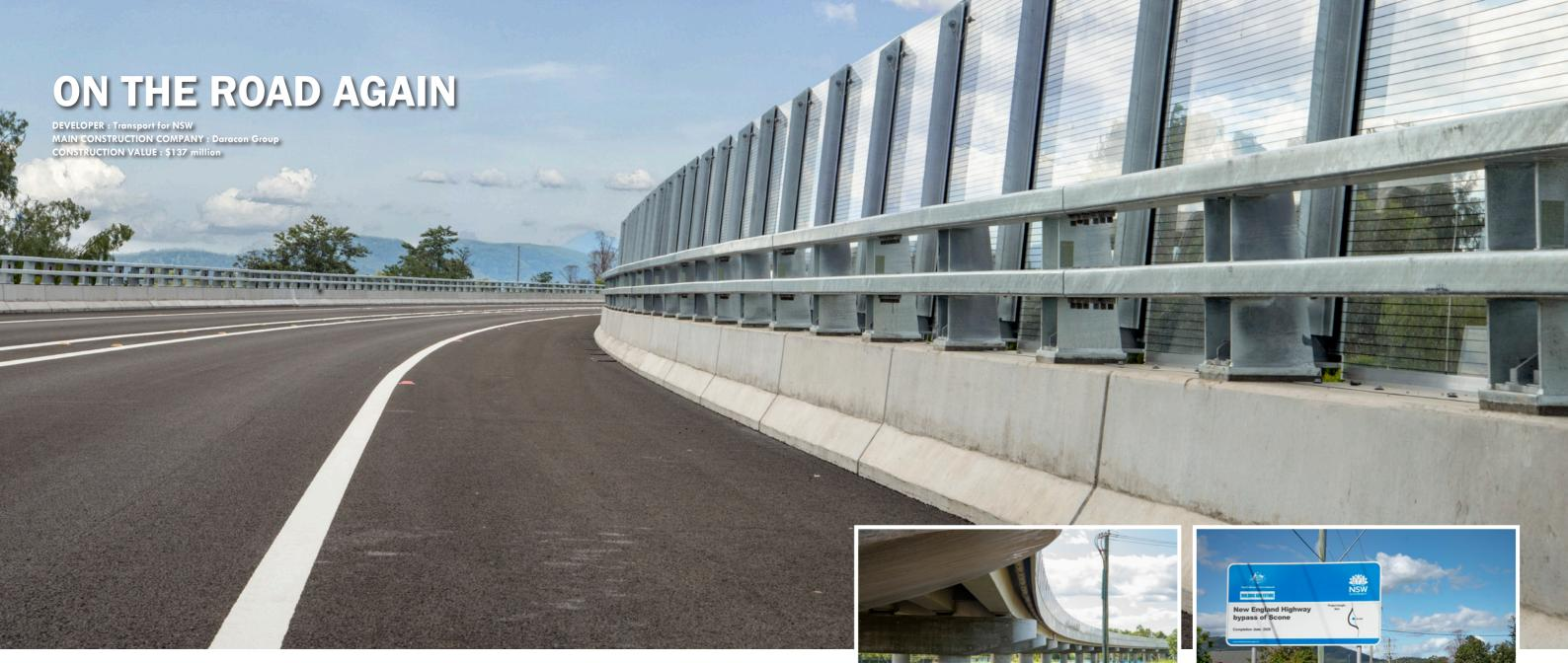
Scone Bypass involved construction of a 5km two-lane bypass which included three new bridges, intersections, associated stormwater drainage, street lights, and road signage. The bypass removes approximately 500 heavy vehicles per day from Kelly Street, and improves road safety and travel times for freight.
