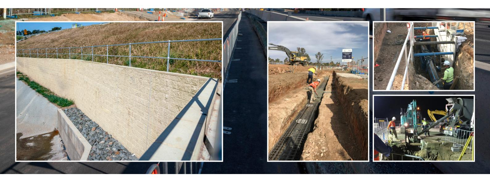
Baines Masonry are a specialist manufacturer of concrete products and supply blocks and pavers in a wide variety of styles and colours. Their product range includes retaining wall systems and a range of accessories, and in 2018, Baines Masonry was contracted to manufacture and supply concrete masonry product for the retaining walls at The Northern Road Upgrade. The blocks supplied were split faced, and pale yellow in colour called 'Appin Stone'.
