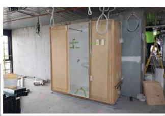
Over the past four years the company has undertaken an extensive development program and has developed their modular bathroom system to incorporate flat packed assembly techniques and has introduced the new Tiled Look finish, taking the product to a new level of feel and finish.
